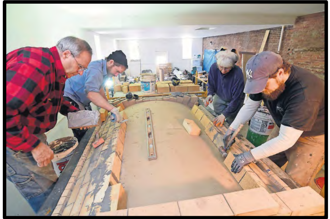
Rebuilding of the wood-fired oven in the historic Rise Up Bakery adjacent to the Old Labor Hall in Barre
